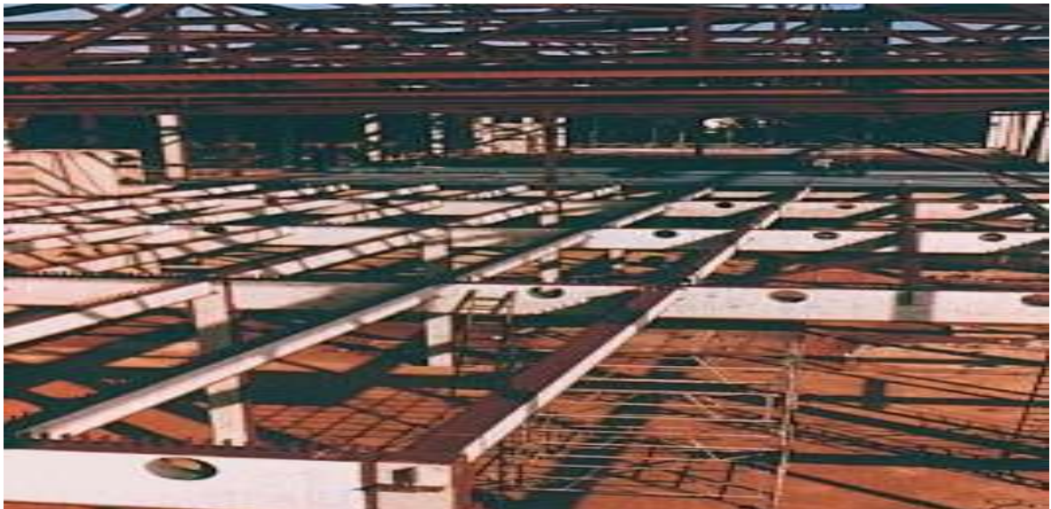
Picture 7 : Partially encased steel sections, for both beams and columns, are an interesting development of the last ten years.
