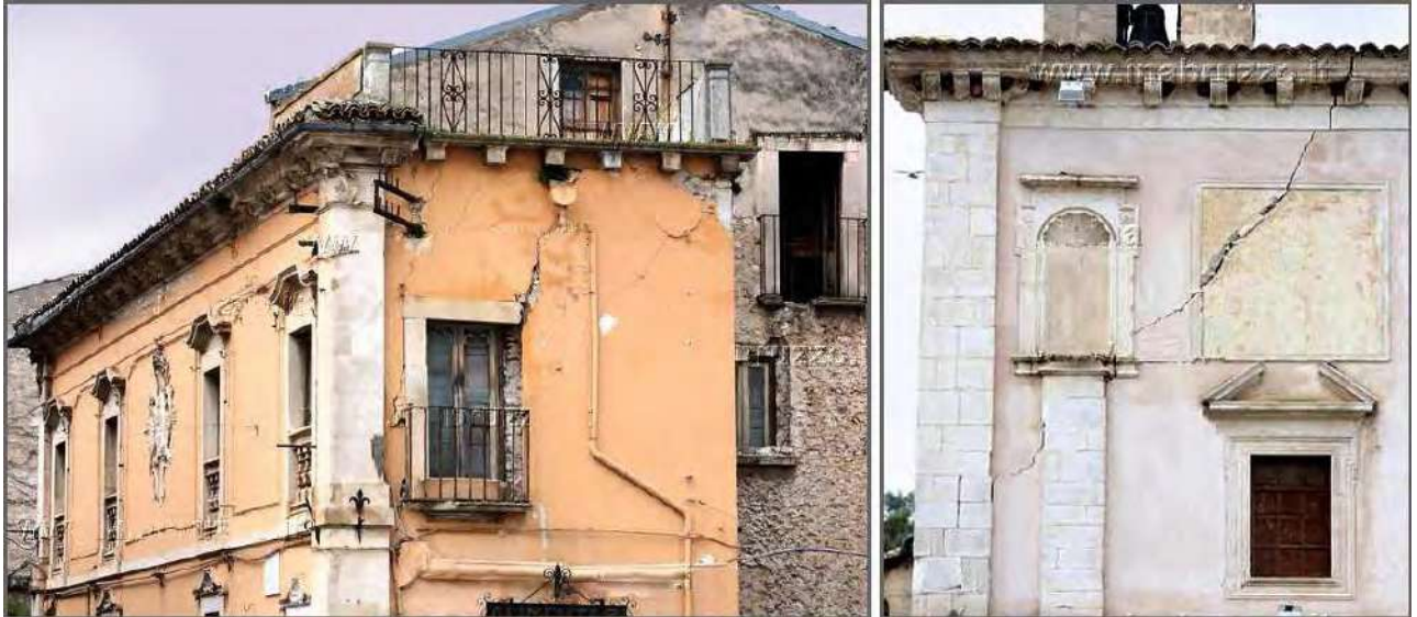
Figure 8.3: Damage in walls due to earthquakes
