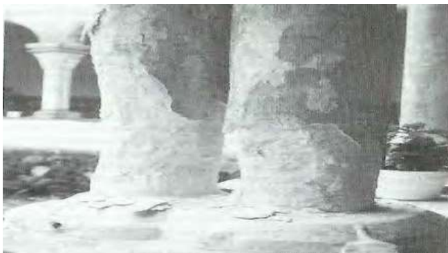
a) Loss of material in columns
