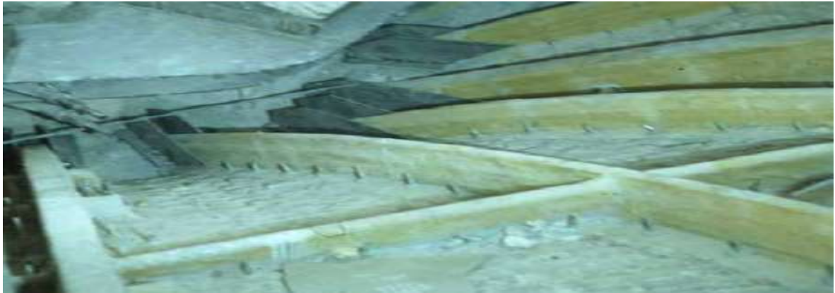
Figure 8.14: Strengthening of masonry vault with timber ribs glued on the extrados
