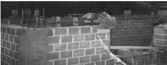
Figure 2. confined masonry construction with hollow block and clay brick
