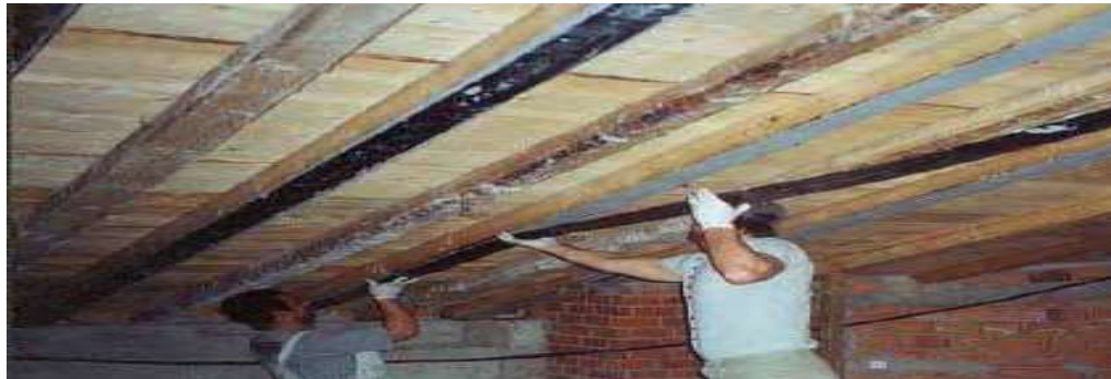
Figure 8.16: Strengthening of timber floor with composites
