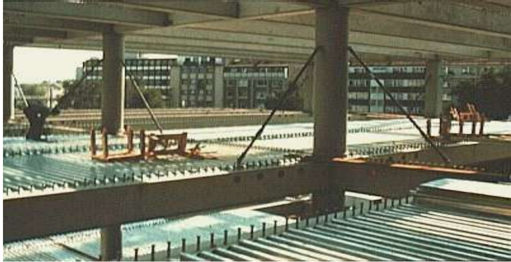
Picture 5 : The usual practice for commercial and industrial buildings is to construct the floors using metal decking which is embossed to provide composite action.
