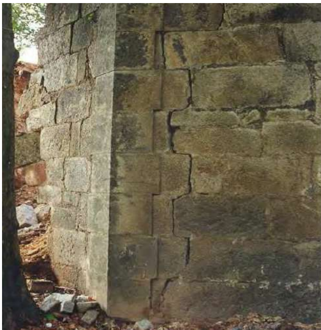
Figure 8.4: Damage in walls due to earth pressure Figure 8.5: Damage in column due to earthquakes
