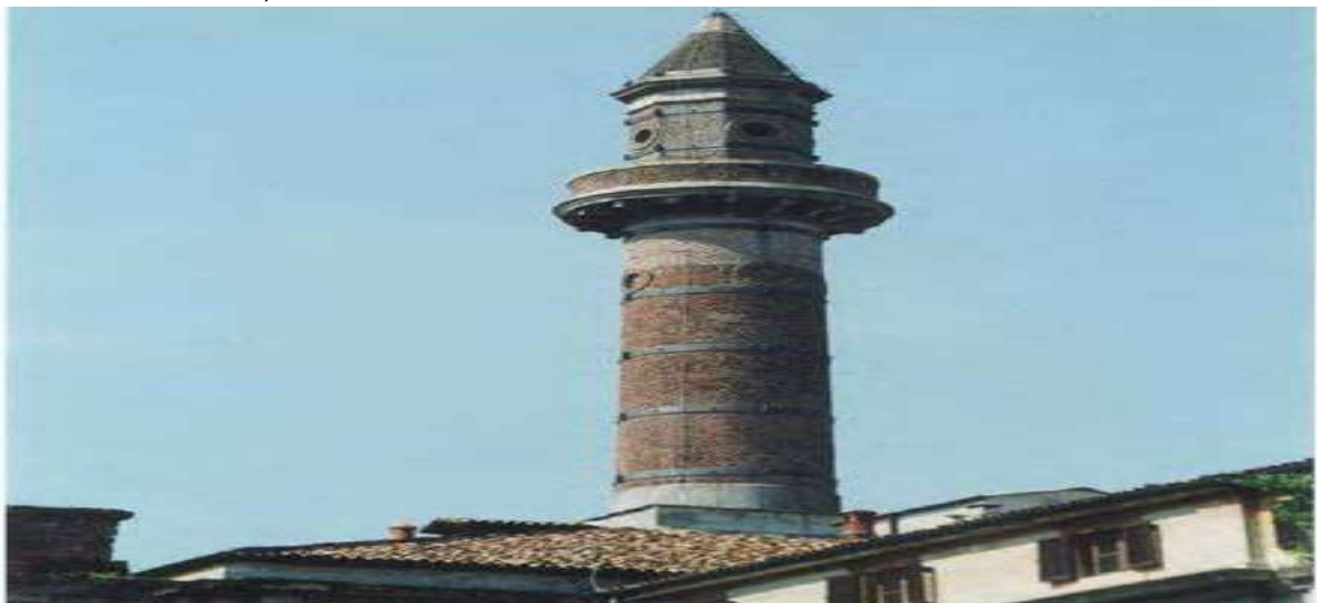
Figure 8.15: Tying of masonry tower with steel strips
