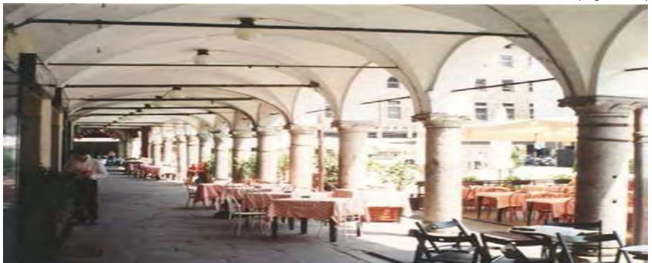
Figure 8.13 Tying of masonry vaults with tie-rods in steel
