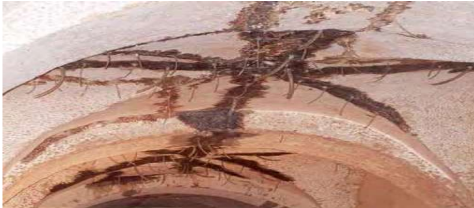
Figure 8.9: Injections of epoxy resins in a masonry vault
