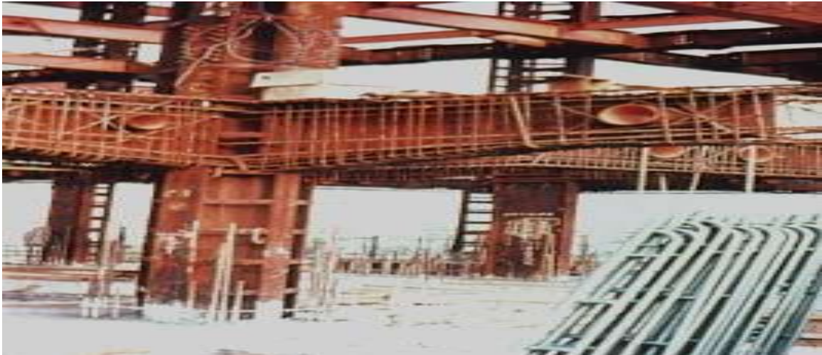
Picture 3 : The combination of concrete cores, steel frame and composite floor construction has become the standard method for multi-storey construction in several countries.
