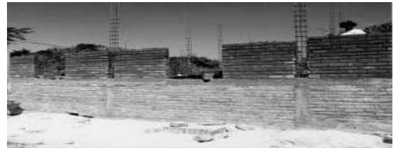
Figure 2. confined masonry construction with hollow block and clay brick
