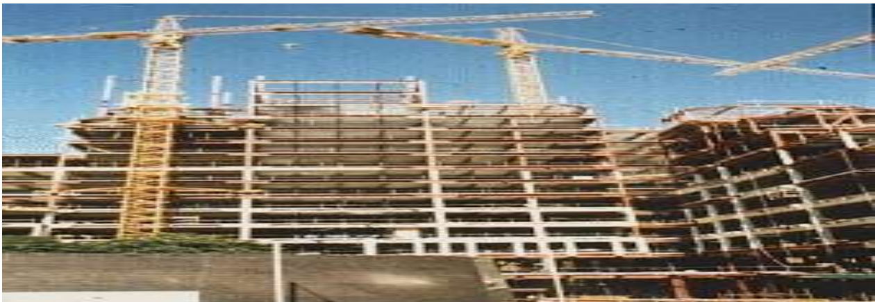
Picture 1 : Typical composite multi-storey steel-framed building during construction - a commercial building in London.
