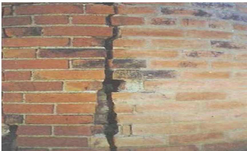
Figure 8.7: Vertical cracking in a masonry chimney
