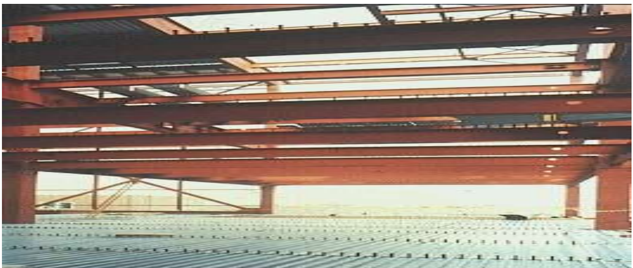
Picture 2 : Typical composite multi-storey steel-framed building during execution - a factory building for the car industry in Germany.
