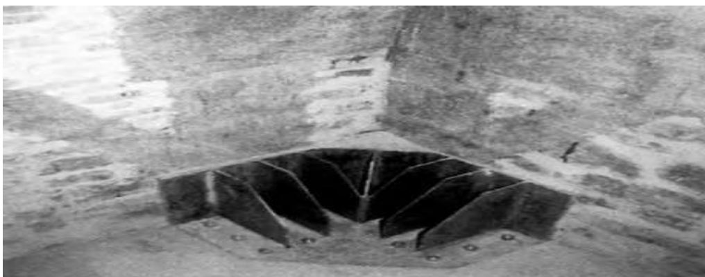
Figure 8.20: Steel device to connect a wooden floor with walls integrating wooden elements
