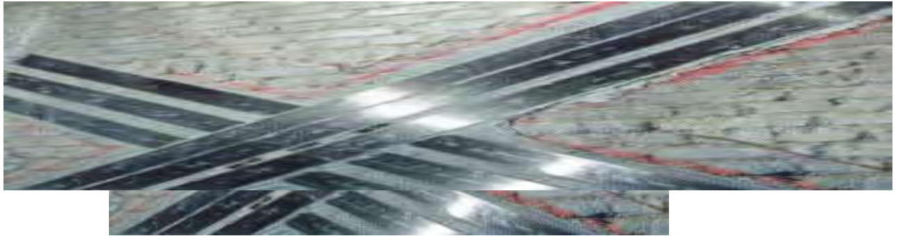
Figure 8.12: Strengthening of a masonry wall with glued CFRP strips
