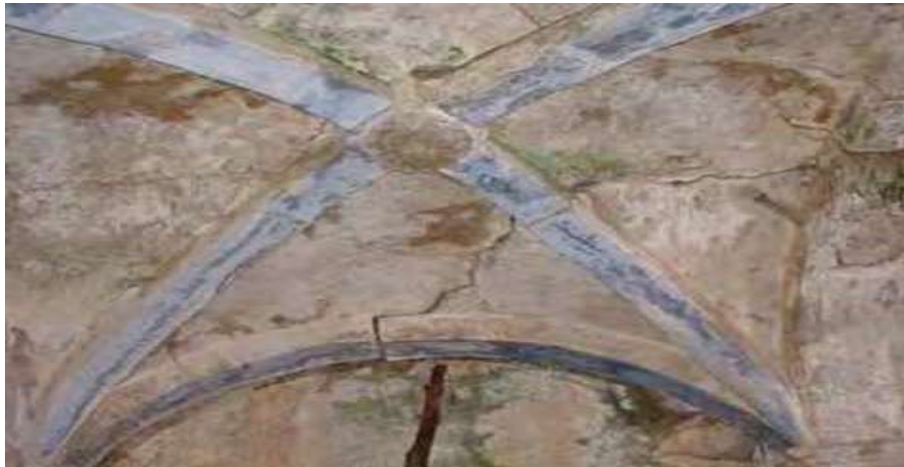
Figure 8.6: Cracks in a masonry vault
