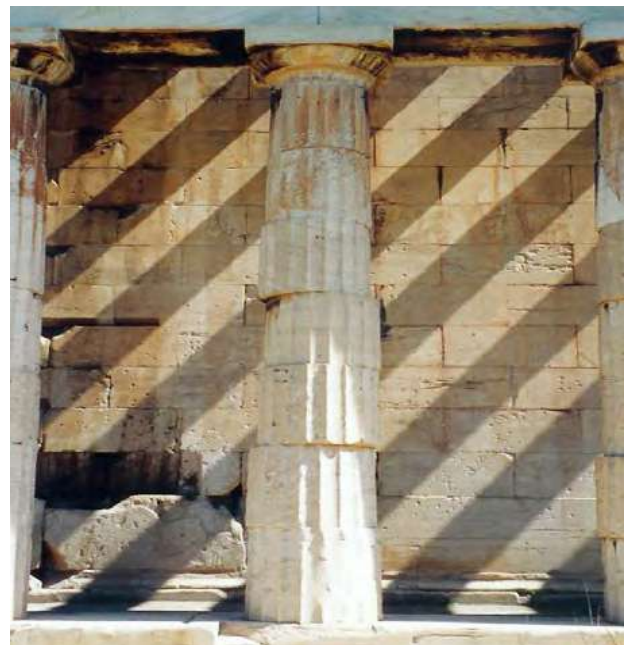
Figure 8.4: Damage in walls due to earth pressure Figure 8.5: Damage in column due to earthquakes
